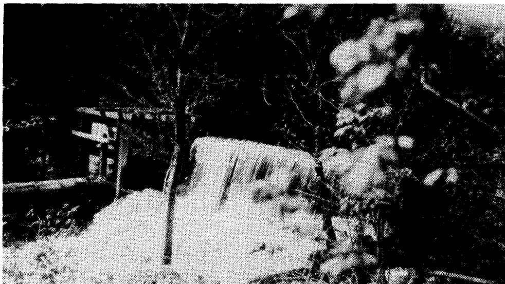
The dam behind the sawmill. The wooden pipe on the left carried in the water power which drove the mill.
